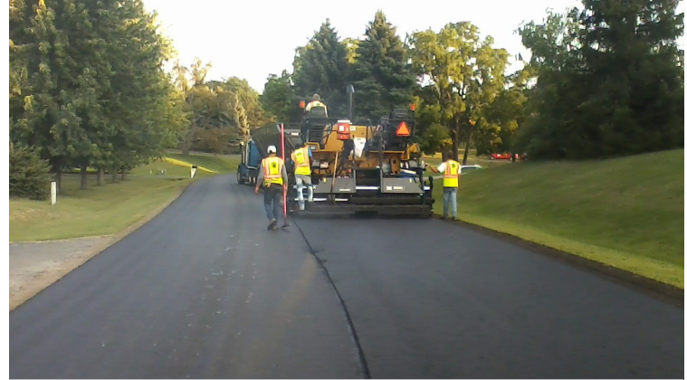
Contractors paving a subdivision, funded by a SAD
